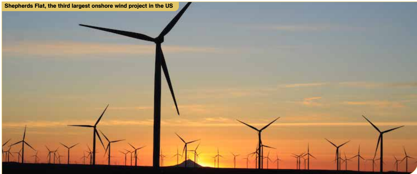
Shepherds Flat, the third largest onshore wind project in the US
